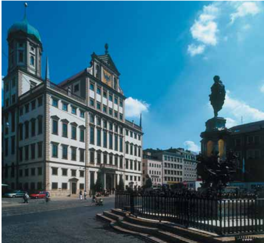
Augsburg Town Hall painted with silicate paint, after 20 years' service life
