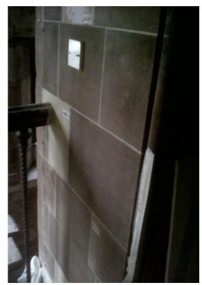
New sections of stonework at Ruyton Manor in Shropshire were clearly very different to the original and were blended using Design Lasur.
