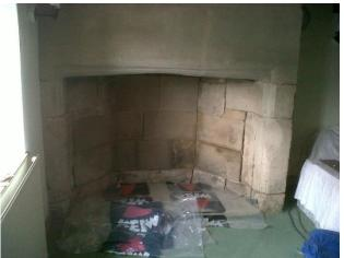
Fireplace stone repairs, colour matched and blended to create a natural stone finish which matches the rest of the stonework.
