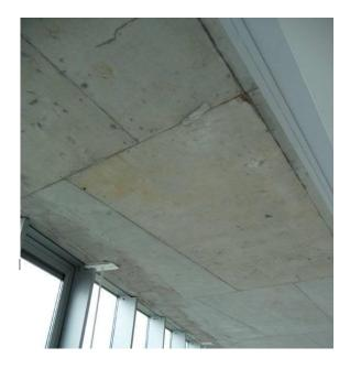
Soffit after KEIM Concretal Lasur applied
