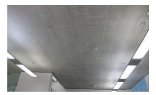
The aim of specifying visual concrete is to achieve a natural, high quality concrete appearance and where necessary KEIM Concretal Lasur can be employed to help achieve this.
