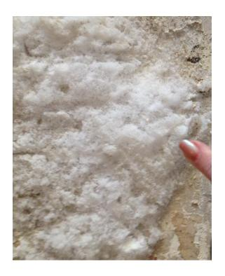
It is common in older buildings for soluble efflorescent salts to be present within the masonry. Mineral substrates contain water in which salts can be dissolved and, as drying and evaporation occurs, this causes the salts to crystallise out, producing white crystals known as efflorescence on the surface. KEIM Mineral Paints offer two primers which, if used appropriately, can significantly help to slow the egression of such salts.
