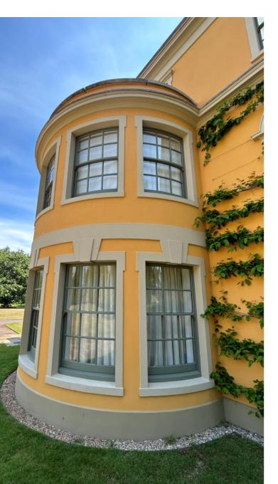
Polymer and acrylic-based repair materials are unsuitable for use with mineral paints, therefore minor cracking and repair work was completed using KEIM Spachtel, a ready-mixed and easy-touse paste filler with mineral fibres.
