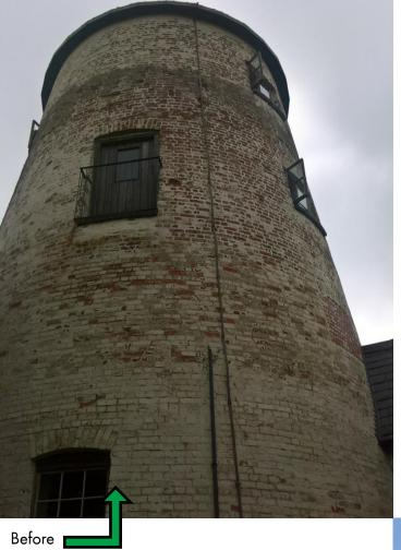
The exterior brickwork of the windmill was patchy and flaking after using limewash.
