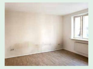
Visible mould after water damage is often only the tip of the iceberg. Microbiological analysis is therefore advisable prior to restoration. This provides the basis for developing and implementing a suitable mould remediation concept. Experts generally advise against using fungicides indoors.
