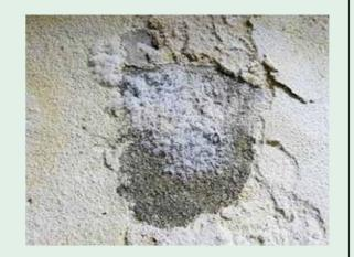
If water penetrates the masonry, salts are often brought to the surface. These salts recrystallise and cause "efflorescence". The result is unsightly, usually white or yellowish stains on wallpaper or render. Efflorescence and crystallisation cause spalling.
