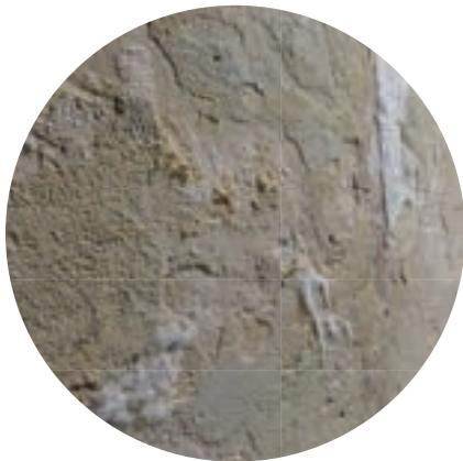
Spalling and salt efflorescences; high salt pressure
