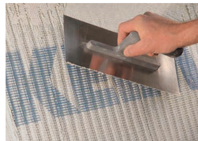
2. Positioning of glass fibre mesh
