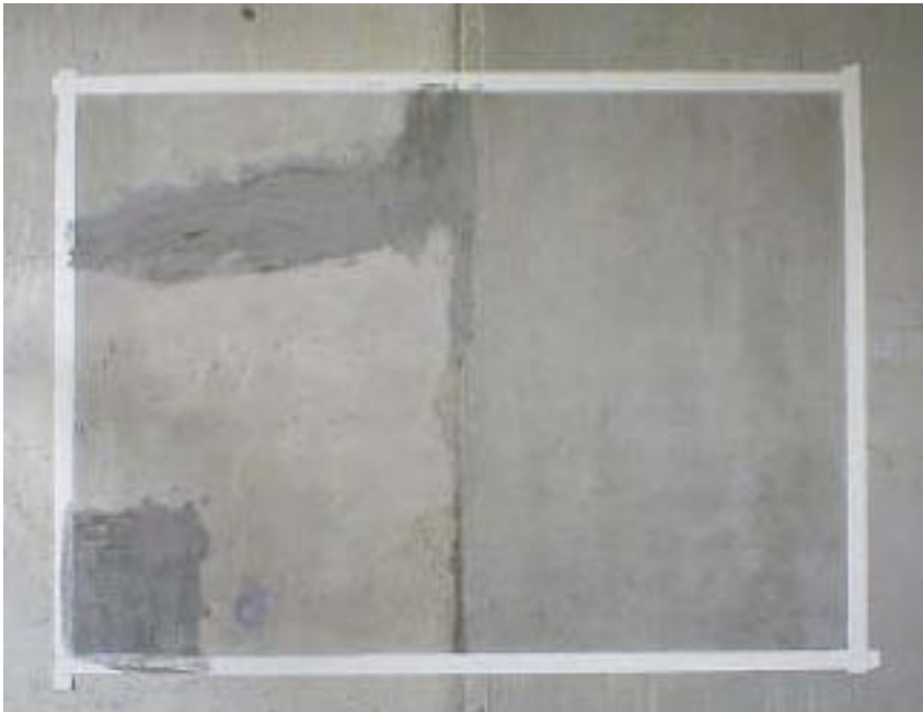
Typical on site repairs and variations
