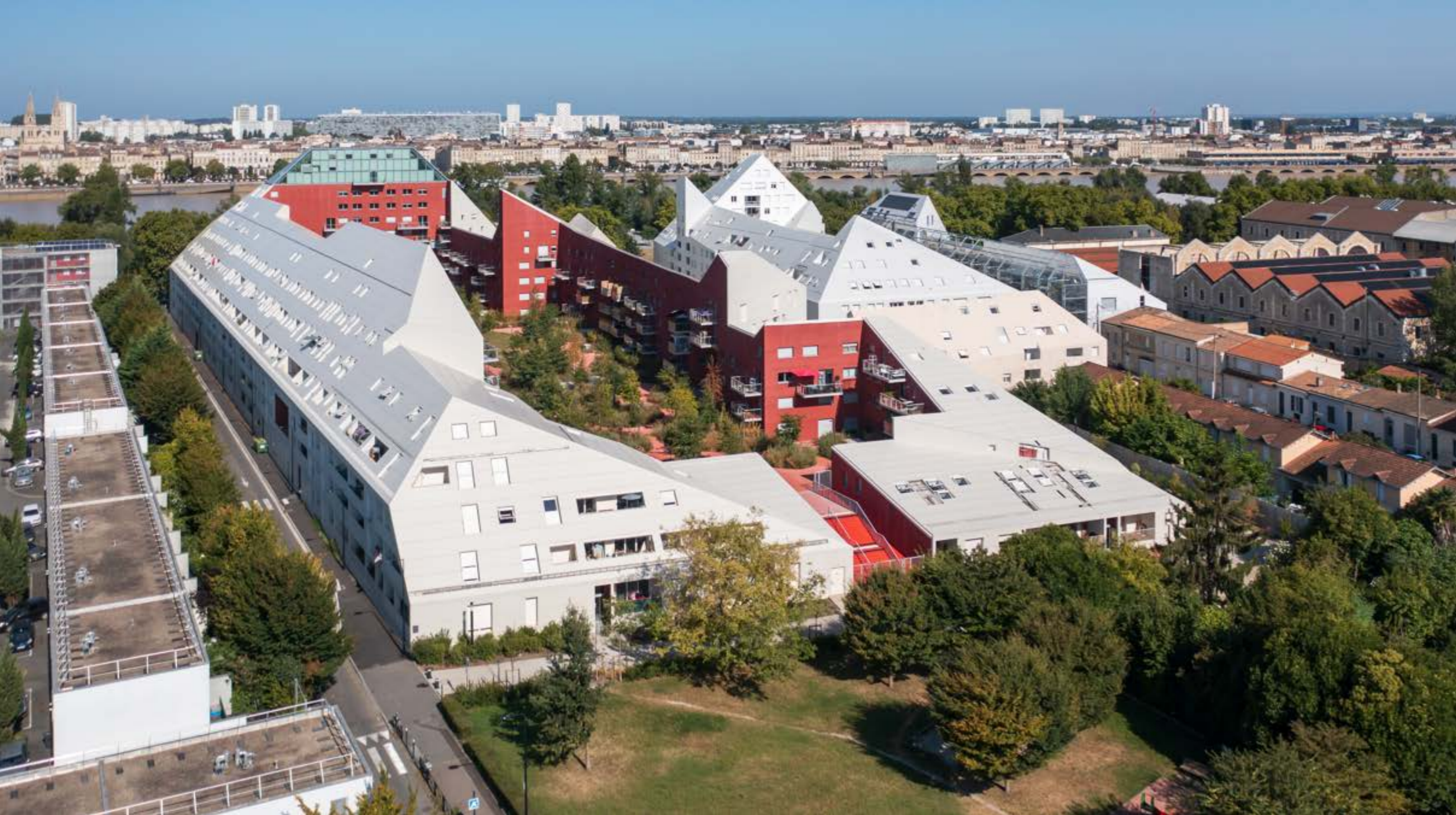
White ceramic panels cover the walls and roofs facing the road, while the façade to the inner courtyard is covered with ruby-coloured stucco.
