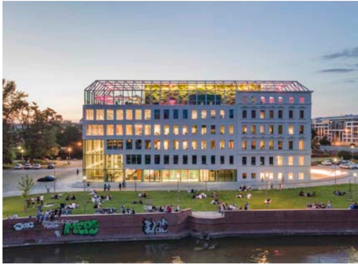
The only building on Stodowa Island to survive World War 2.
