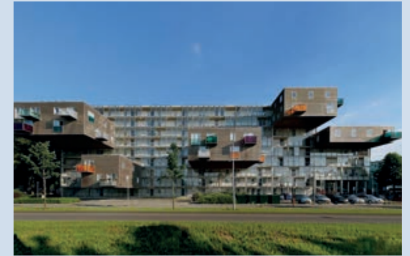
WoZoCo, Amsterdam, 1997 The house for elderly residents has whole units cantilevered from the north façade. As a result, there is less shading of the neighbouring buildings while optimum use is made of the available land without sealing the ground.
