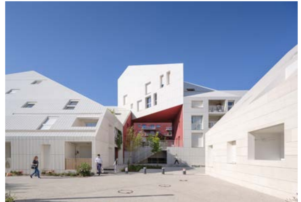
White ceramic panels cover the walls and roofs facing the road, while the façade to the inner courtyard is covered with ruby-coloured stucco.
