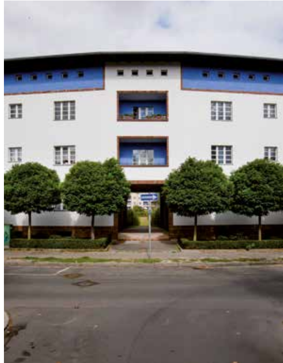
Photo above and left: The Hufeisensiedlung („Horseshoe Estate“) in Berlin – icon of modern urban planning – designed by architects Bruno Taut and Martin Wagner together with garden architect Leberecht Migge.
