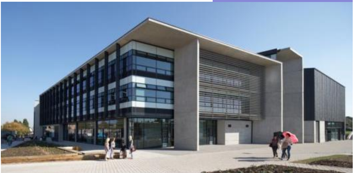
Loughborough University, Faculty Building & Business School 2011 - KEIM Concretal Lasur
