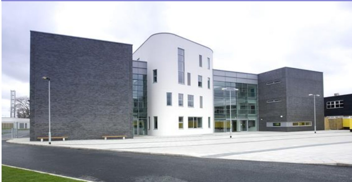
Loxford School of Science & Technology, Ilford 2009 – KEIM Concretal W
