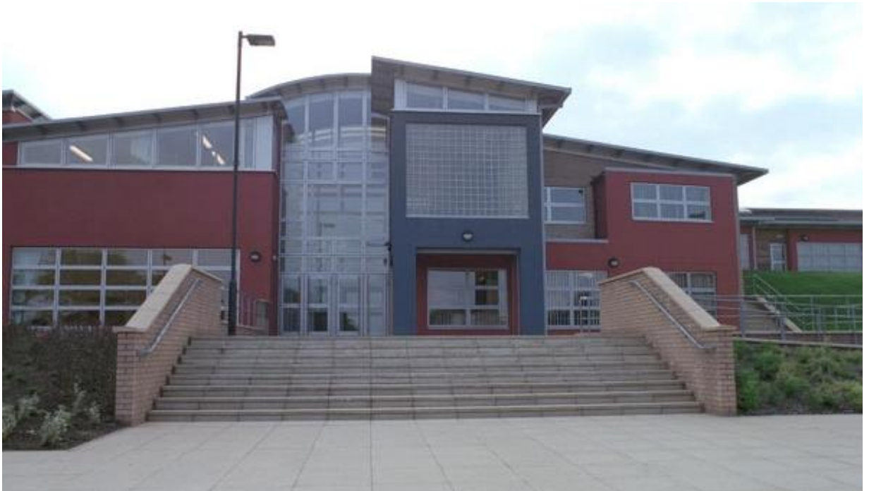
Greenfield County Primary School, Flintshire 2003 - KEIM Universal Render & KEIM Granital (KEIM Ecosil-ME Internal)
