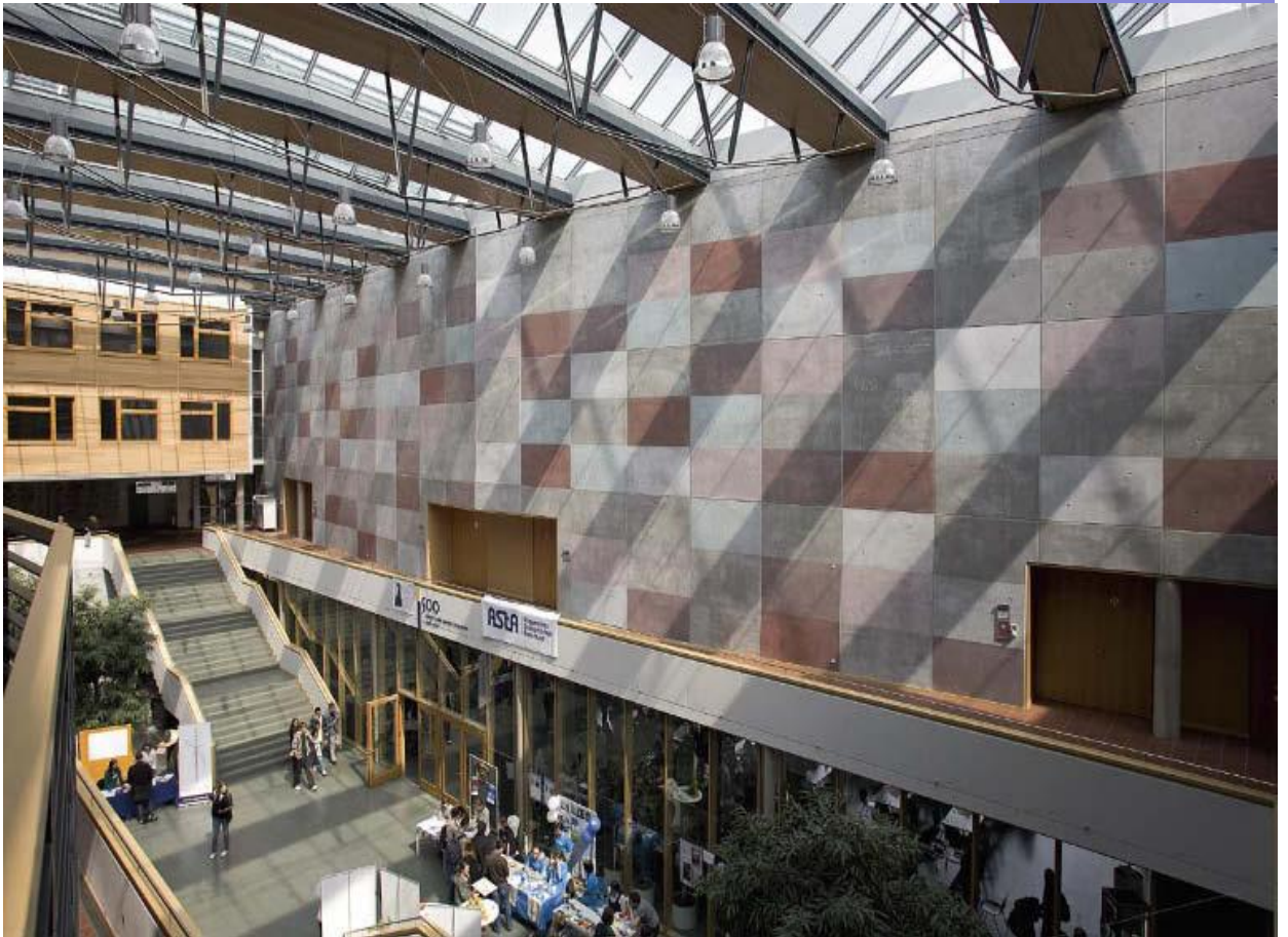
Frankfurt University Auditorium - KEIM Concretal Lasur
