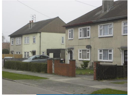
Barfield Road, York - Before
